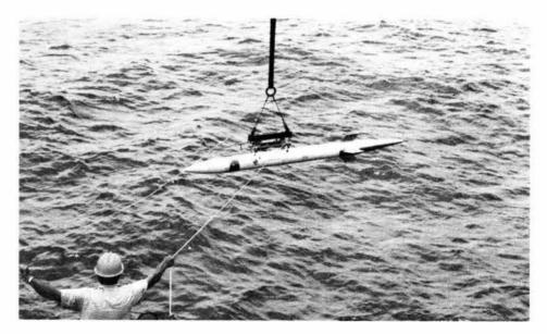
READY FOR FREE-FALL into the seabed off the California coast, this Instumented Seabed Penetrator carried an Explosive Acoustic Telemeter that allowed computation of the impact velocity and penetration depth after a fall through 1700 meters (more than a mile) of ocean.
